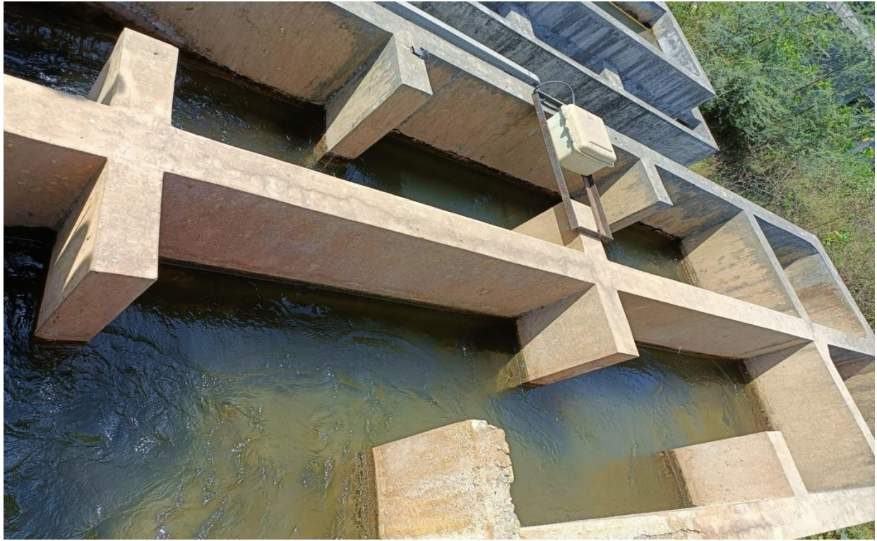
Image 5: Raw Water collection system from Intake
