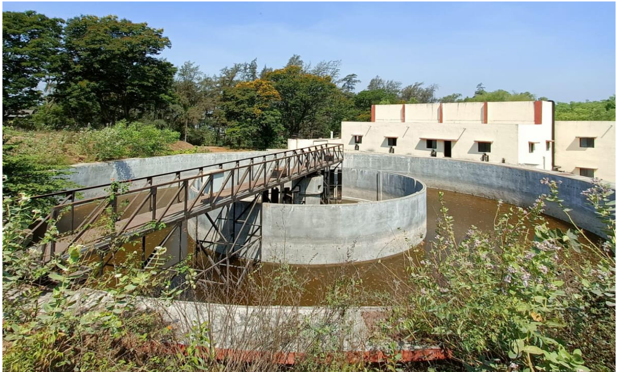
Image 8: Clariflocculator (under construction)
