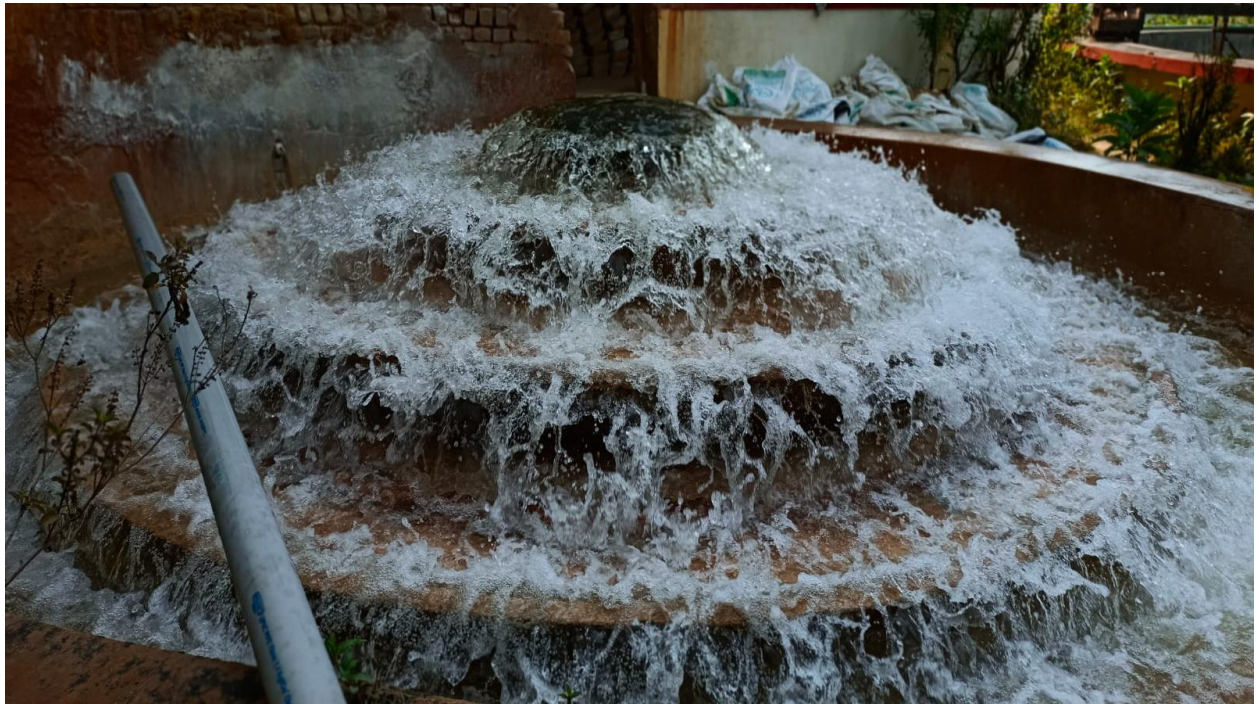
Image 4: Raw Water collection system from Intake
