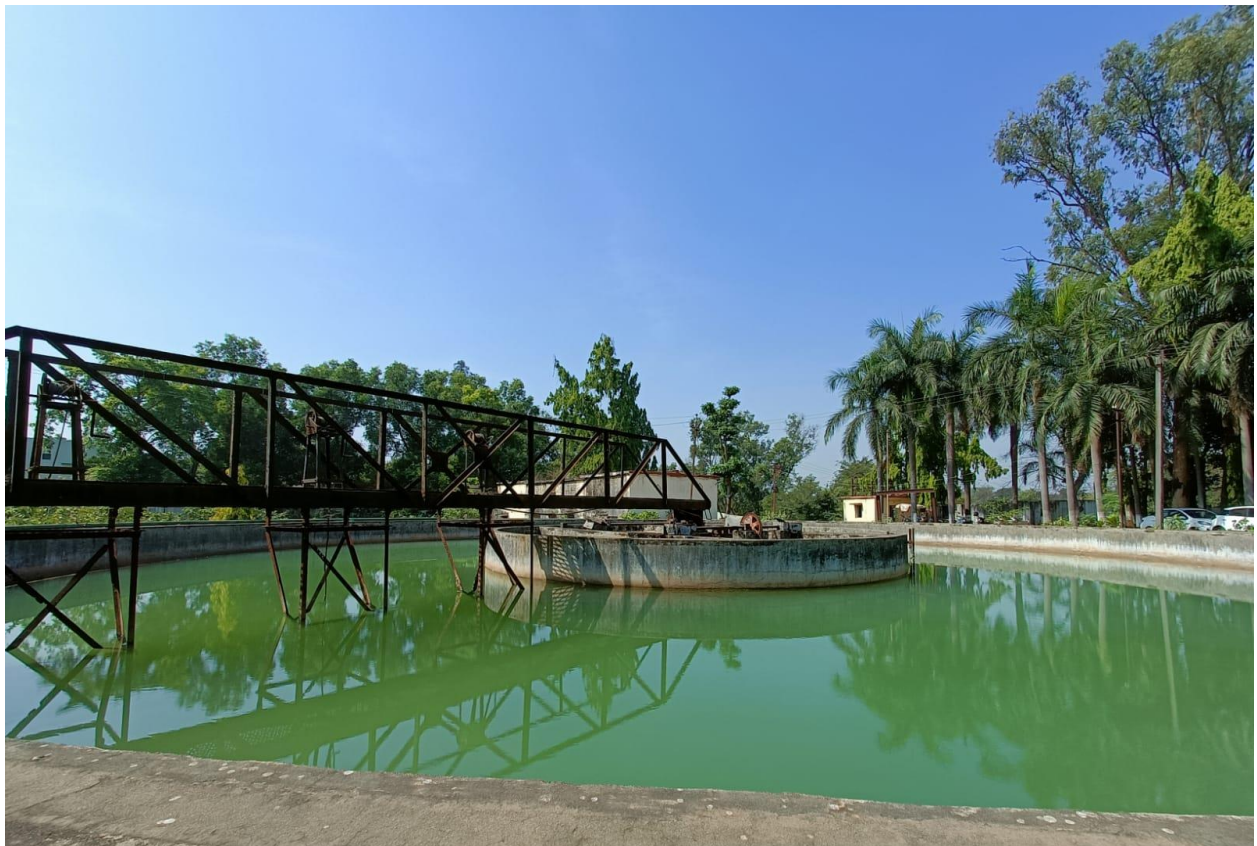
Image 6: Clariflocculator (in working)
